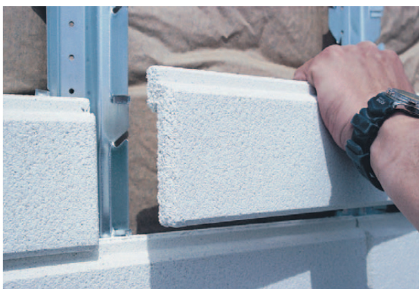
Marmoroc during fitting
