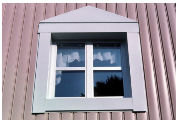
Snaploc, example of window detail
