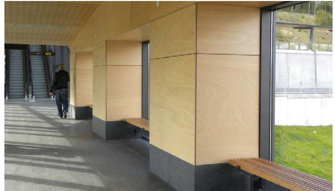
Travel centre Örnsköldsvik, walls and ceiling
