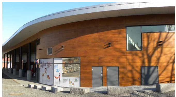
Curved façade, Landvetter travel centre
